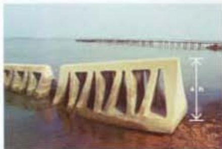
Beach Prisms work by reducing the amount of energy in incoming waves before the waves reach the shoreline. Waves pass through the specially designed slots.
