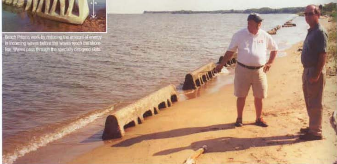
Louis Marusik, General Manager at Smith-Carolina, and Jay McKenna, Regional Sales Manager, at the Terrapin Nature Area. Only the top of the prisms show, indicating the amount of sand that has been accumulated on that beach.
